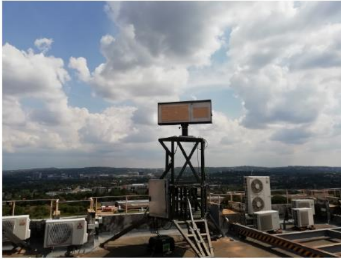
Figure 4.1: Radar on top of the roof of building 44 at CSIR's main campus in Pretoria [34].
