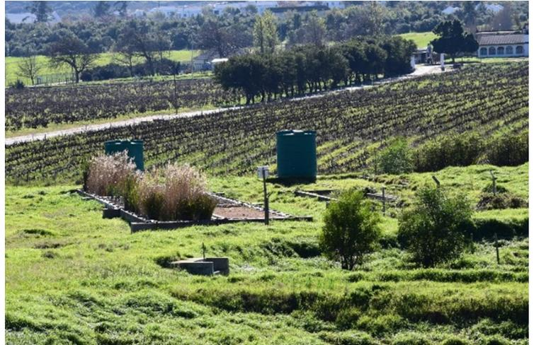
*Biofiltration treatment cells that are used for polishing and cleaning polluted water from the informal settlement*
