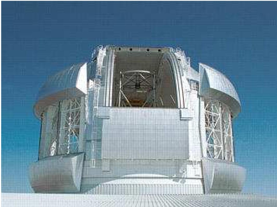
Figure 8: The Gemini (South) telescope showing the large vents opened. Note the much greater area of these designed vents compared to the “modification” fittings on the other CTIO telescopes.
