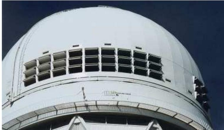
Figure 7: Close up of air flow vents on the CTIO 4m telescope.
