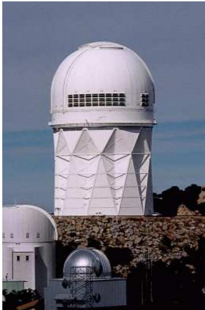
Figure 6: Air flow vents on the CTIO 4m telescope.
