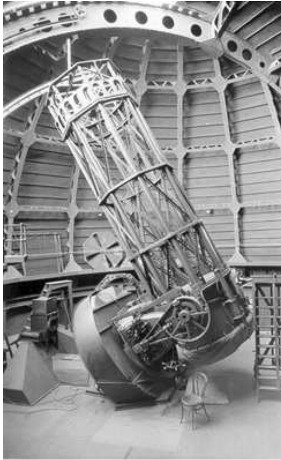
Figure 39: Mt Wilson Observatory 60-inch (1.5m) telescope. (Polar disc mount).
