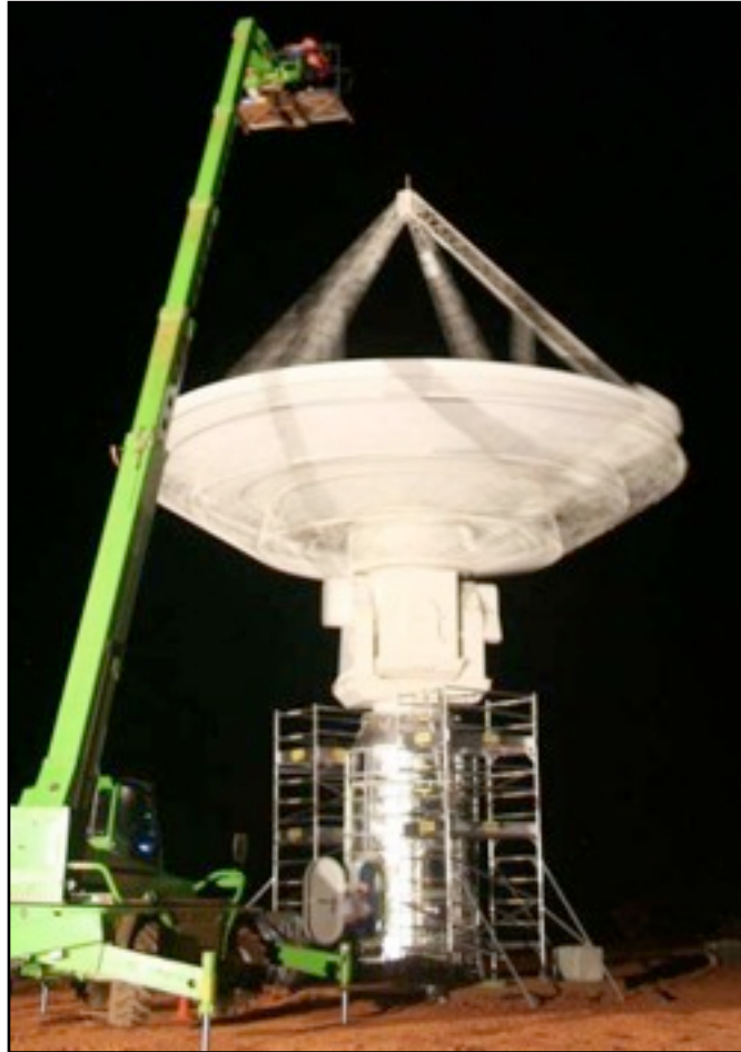
▲ Installation of the receiver housing
