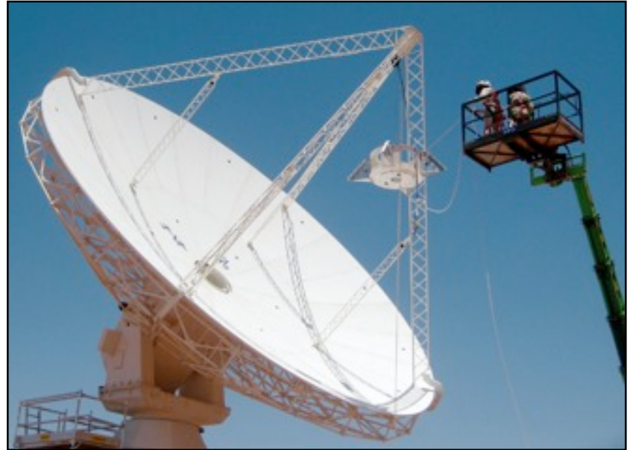
▲ Installation of the receiver housing
