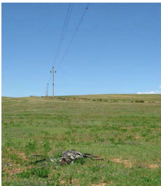
A Blue Crane Anthropoides paradiseus carcass under a power line with defective markers designed to reduce bird collisions with the wires. Photo: Jessica Shaw.
