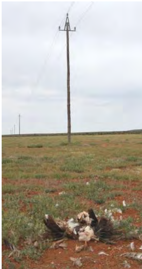
A Ludwig's Bustard killed by low-voltage power lines near Calvinia. (Photo: Maurice Schutgens)
